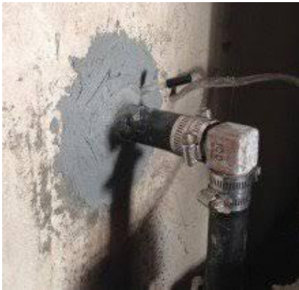
Through a masonry wall
