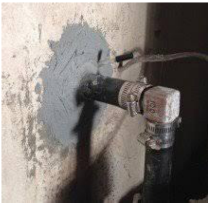
Through a masonry wall
