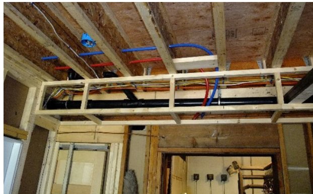
Around raceways and chases that are usually closed with a bump-out
