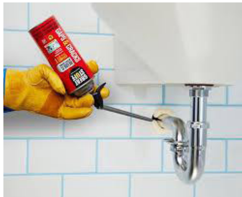
Bathroom pipe penetrations
